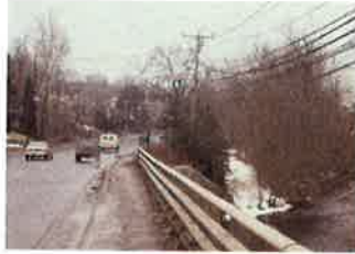
2.99 Long Ridge Road-bridge at crossing with Mill River
