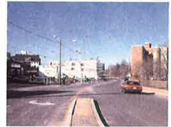
2.44 Washington Blvd. looking north
