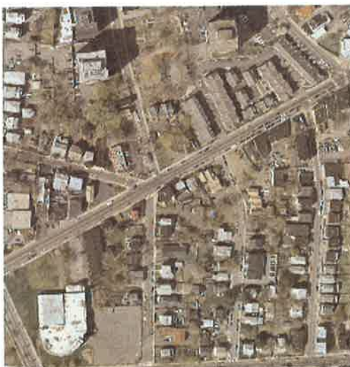
2.35 West Main aerial photograph
