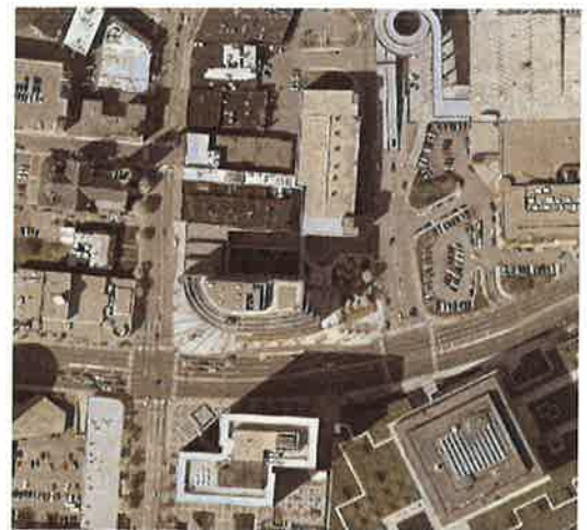
2.64 Tresser Boulevard aerial photograph
