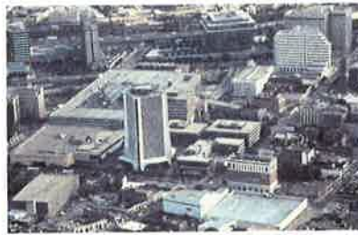
1.26 Aerial photograph of Downtown, showing scale conflicts.
