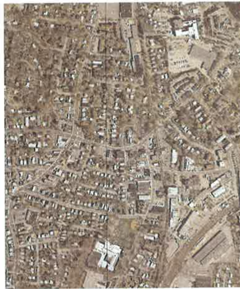
3.16 Glenbrook neighborhood center-aerial photograph
