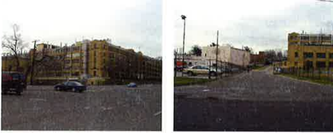
4.30 and 4.31 Photos of existing older buildings
