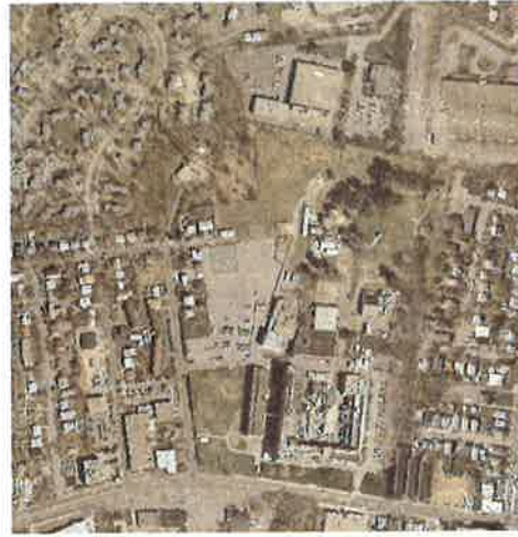
4.37 The industrial campus-aerial photograph
